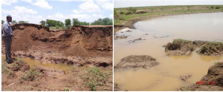
Figure 5.3: Impacts of Allaybaday flash floods: a photo of a broken sand dam in the area due to a recent flash flood 10
